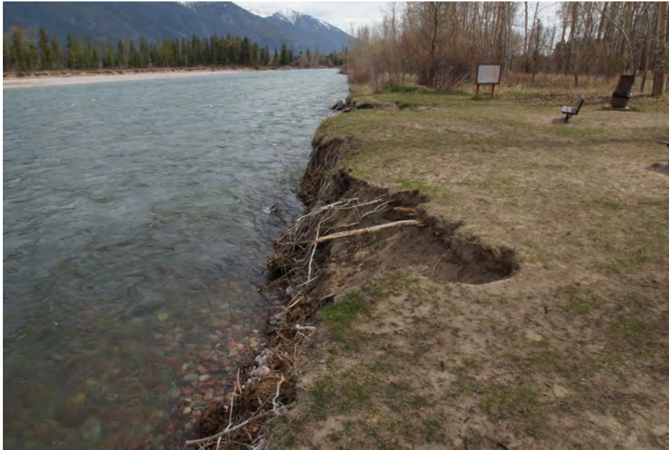
Figure 5. Eroding reach at River's Edge Park.
