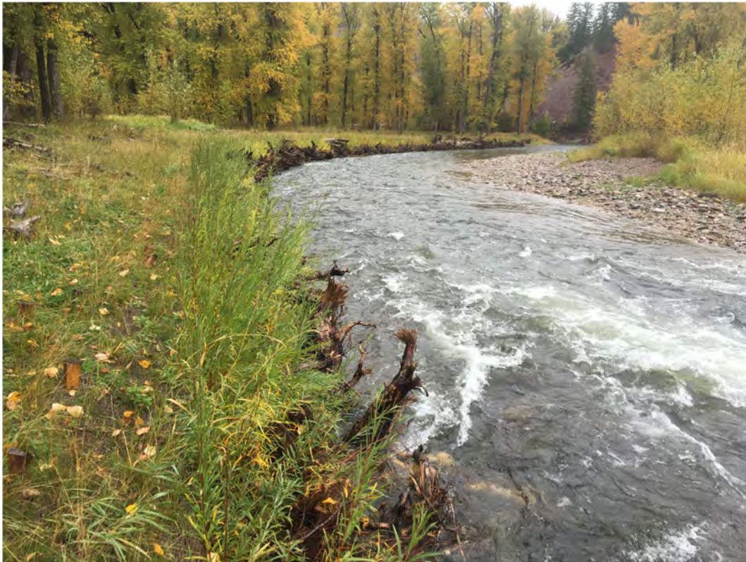
Figure 6. A soft streambank stabilization on Rock Creek, Missoula County.
